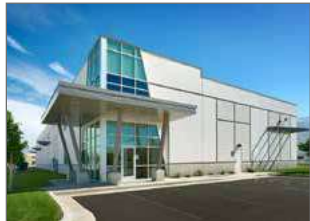
Building entrances should be highly visible with projections for winter design
